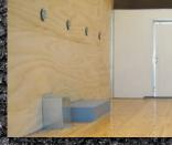
Plywood lining with D-rings
